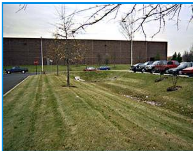
Vegetated swale/filter strip
