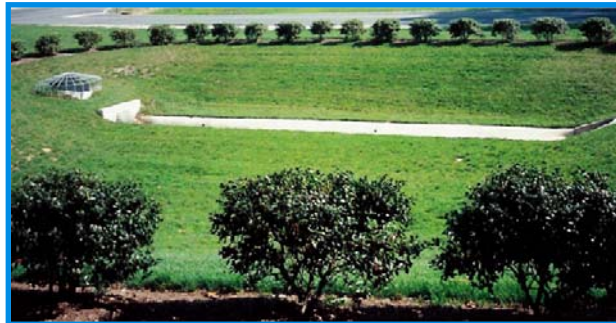
Dry detention pond
