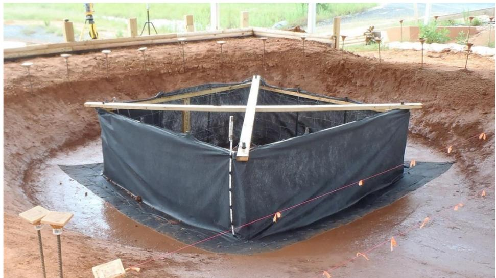
Figure IP-2 Silt Fence Inlet Protection installation showing silt fence, geotextile underlayment, steel T-posts, 2 x 4 bracing, and dewatering device. (Photo courtesy of AU-ESCTF. See Appendix for CAD files)
