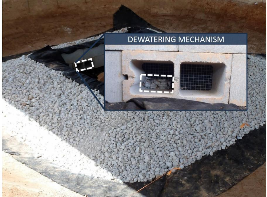
Figure IP-4 Block and Gravel Inlet Protection installation showing dewatering device. (Photo courtesy of AU-ESCTF. See Appendix for CAD files)
