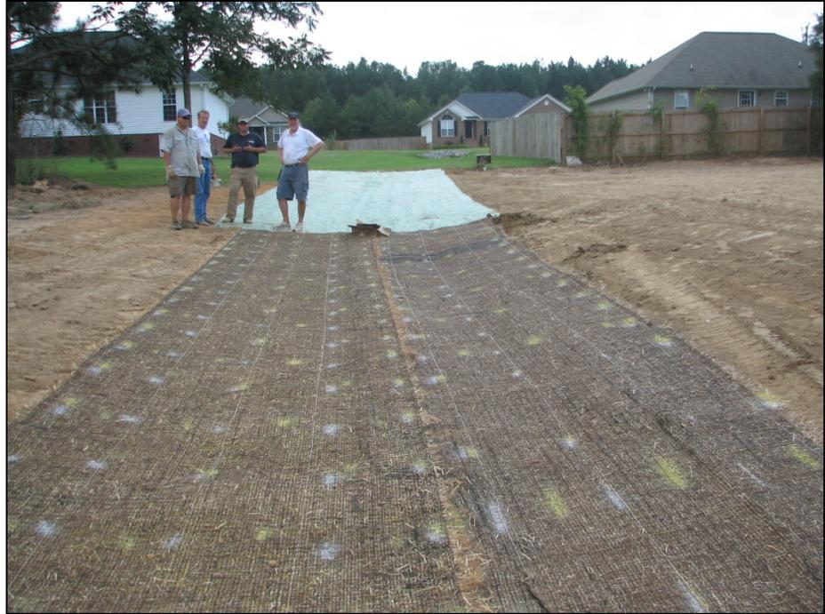
Figure ECB-4 TRM with Pre-Marked Stapling Pattern.
