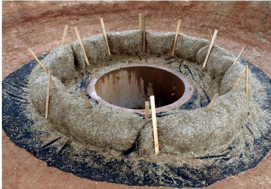
Figure IP-6 Wattle Inlet Protection installation.
