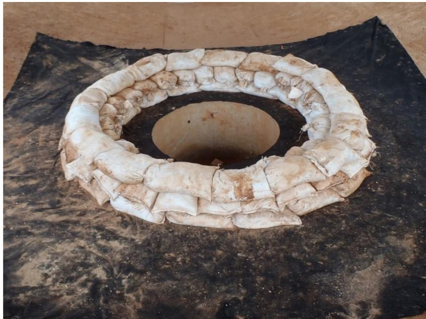
**Figure IP-5 Sand Bag Inlet Protection installation.**
