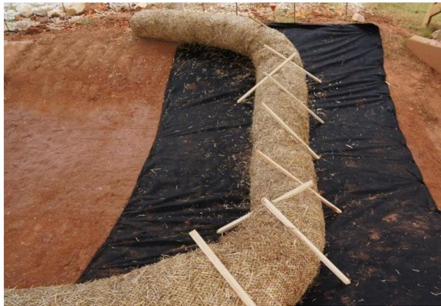
Figure CD-4 Wattle Check Dam (ditch check)
