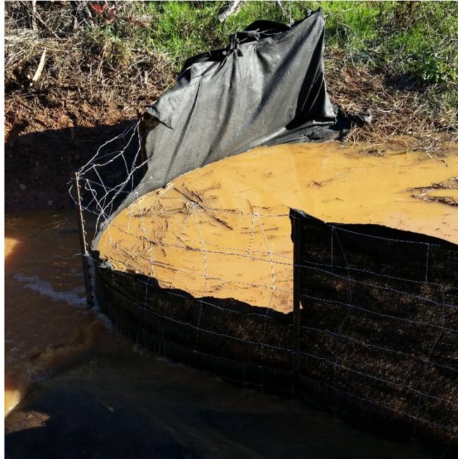
Figure CD-7 Silt Fence Check Dam
