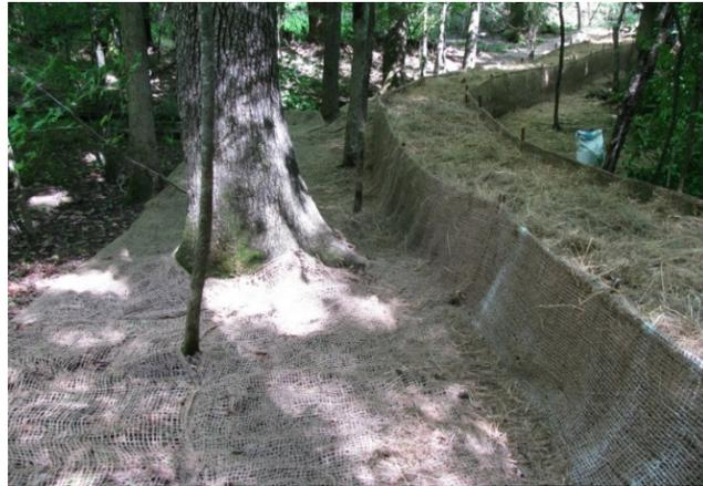
Figure SB-1 Sediment Retention Barrier
