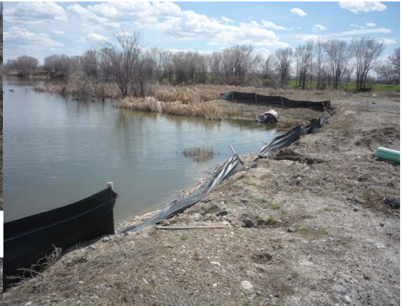
Improperly installed and unmaintained silt fencing.
