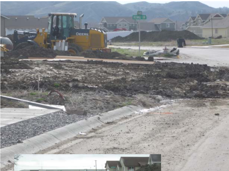
Examples of excessive tracking of mud onto local streets due to lack of access control during construction.
