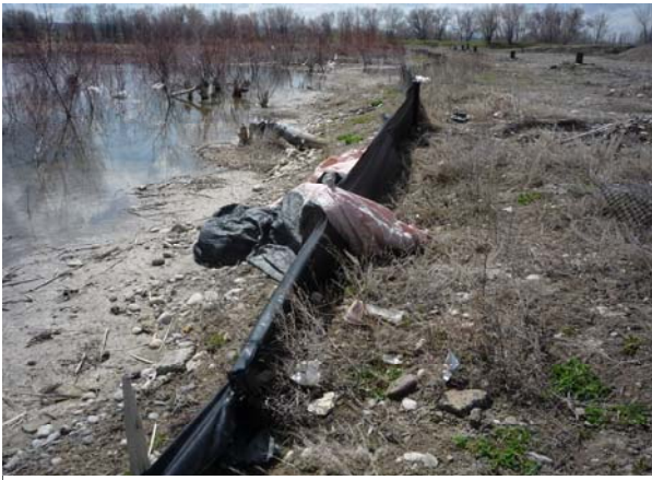
Improperly installed and unmaintained silt fencing.
