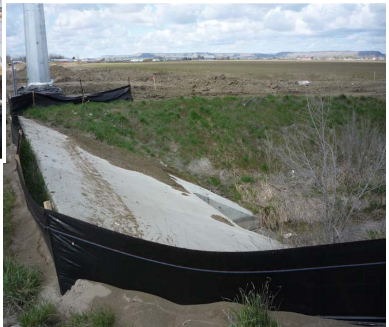
Properly installed silt fencing.
