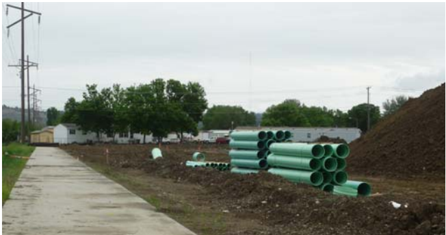
Staged construction on a commercial subdivision. The sidewalk has been constructed and is kept clean during construction activities.
