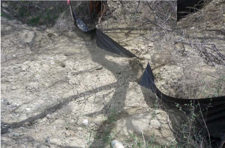
Improperly installed and unmaintained silt fencing.
