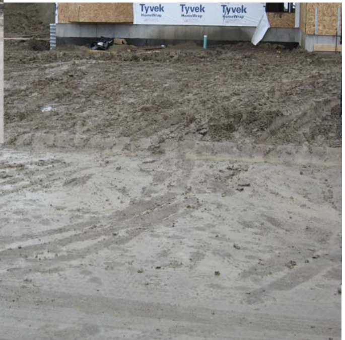
Examples of excessive tracking of mud onto local streets due to lack of access control during construction.
