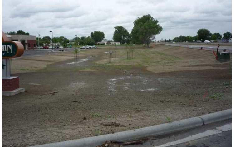
Example of stormwater detention area constructed while property is still under construction.
