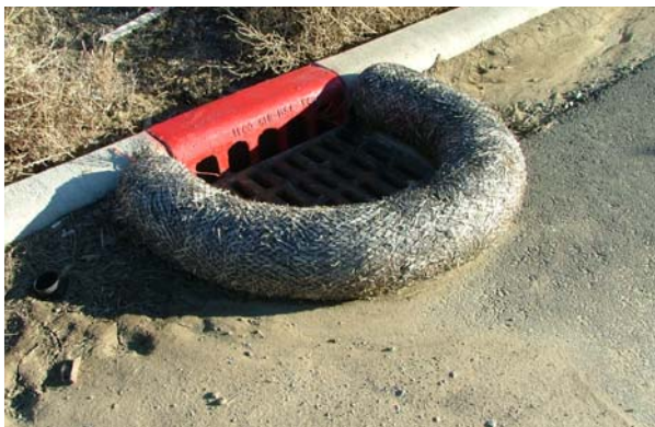
Straw wattle installed at stormwater inlet
