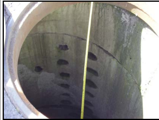
Figure 4.b. Interior of a Dry Well
