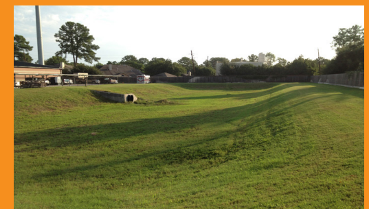
A dry detention pond: Embankments and bottom are grassed to provide erosion protection and stormwater.
