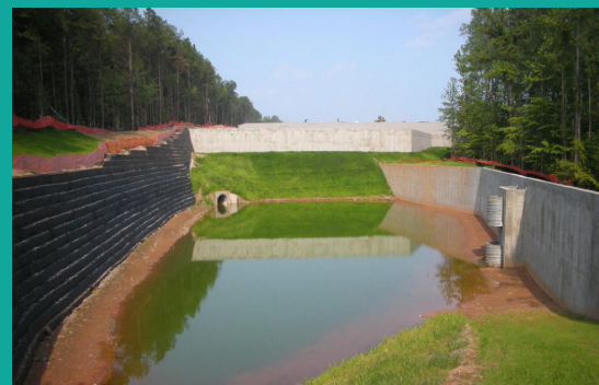
Concrete-walled dry detention pond with earthen bottom: Concrete sides provide erosion protection. The grass is well maintained with no unwanted plants. The bottom of this pond dries between storm events and indicates a well-designed and maintained detention facility.
