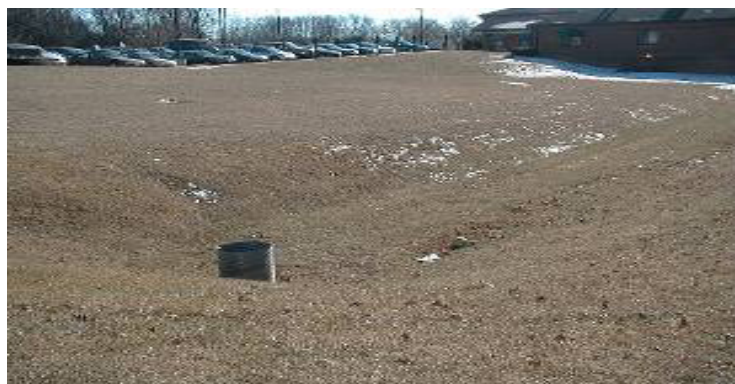
Infiltration basins are designed to collect stormwater from impervious areas and provide pollutant removal benefits through detention and filtration
