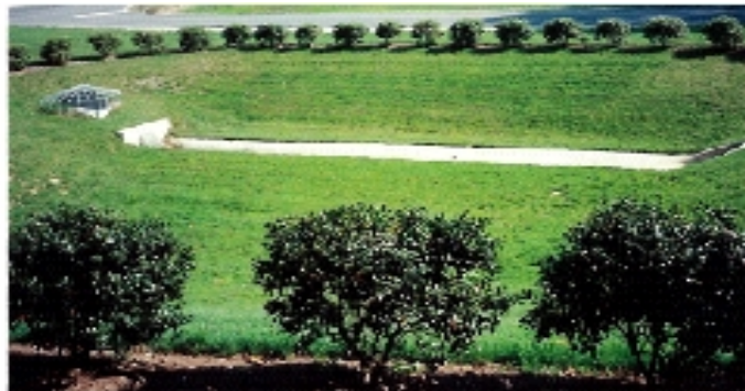
Photo of a dry detention pond designed to temporarily detain runoff during storm events
