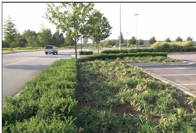
Figure 1.3.2-26 Parking Lot Stormwater “Island”
