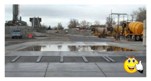
**Figure IC-8a**. The photograph above demonstrates good storm water management practices at a fixed facility. A tire wash at a local concrete ready-mix operation reduces track out of sediment and concrete waste onto paved roadways. (Source: Sparks Environmental Control)
