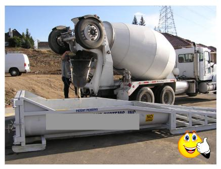
**Figure IC-8d.** The photograph above demonstrates good storm water management practices at a construction site. Concrete washout is contained in a portable washout system and the waste materials are recycled (Source: Concrete Washout Systems, Inc.).
