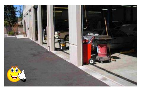
**Figure IC-1d**. The photograph above demonstrates good storm water management practices. A trench drain located near the edge of the covered working area of this vehicle repair facility prevents spills and wash water from draining onto the pavement and entering the storm drain system. (Source: U.S. EPA)
