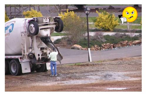
**Figure IC-8b.** The photograph above demonstrates poor storm water management practices at a construction site by a mobile concrete ready-mix operation. Concrete washout should **never** be discharged onto the ground surface, into landscaped areas or into the storm drain system (Source: Concrete Washout Systems, Inc.).
