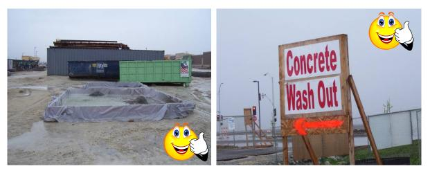
**Figure IC-8c.** The photographs above demonstrate good storm water management practices at a construction site. A dedicated signed concrete washout area is provided in waterproof containment system and the waste materials are recycled (Source: Kennedy/Jenks).
