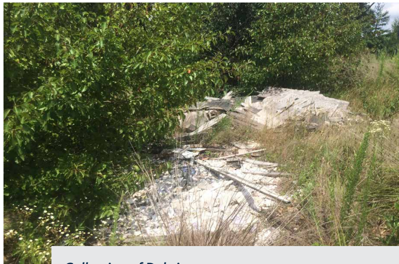
Collection of Debris, Inadequate Maintenance
