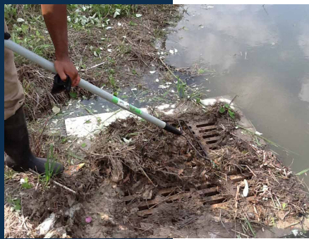
Figure 9: Stormwater Maintenance; structure maintenance and inspection
