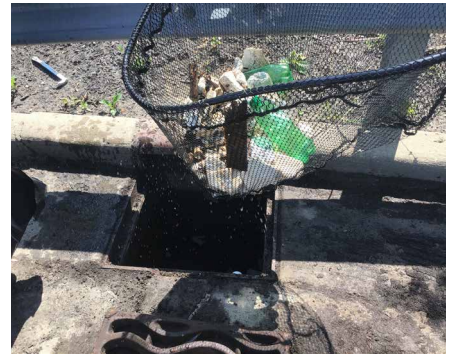
Figure 4: Underground system cleaning and filter replacement
