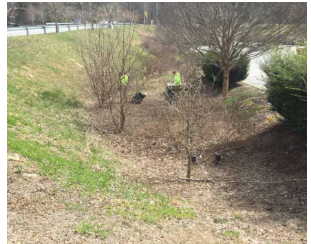
Figure 8: Stormwater Maintenance; mowing, trash control, aerate and overseed
