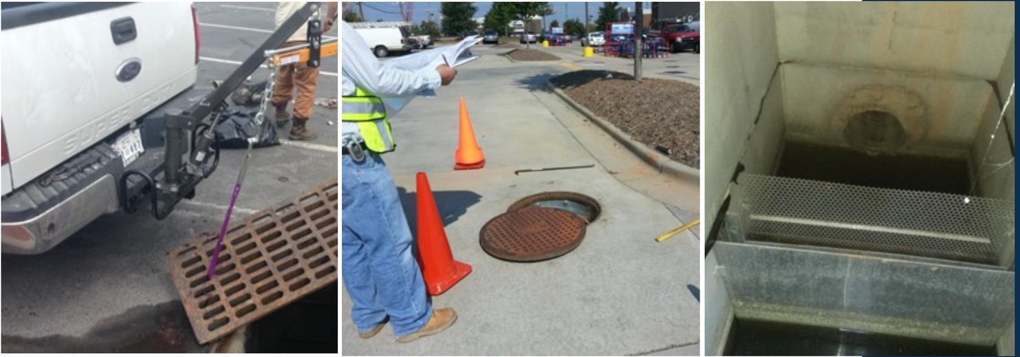
Removing manhole covers and inlet grates for access and observation of sumps and proprietary devices; confined space entry
