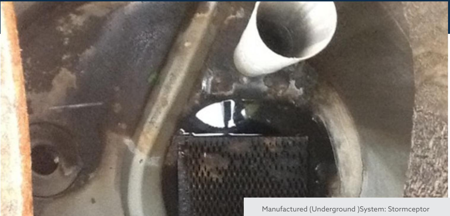
Manufactured (Underground )System: Stormceptor
