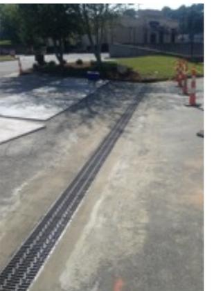
Trench drain installation
