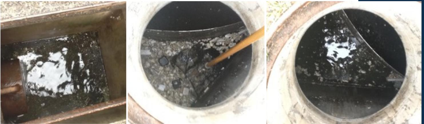
Catch basin sump cleanout; underground detention trash removal
