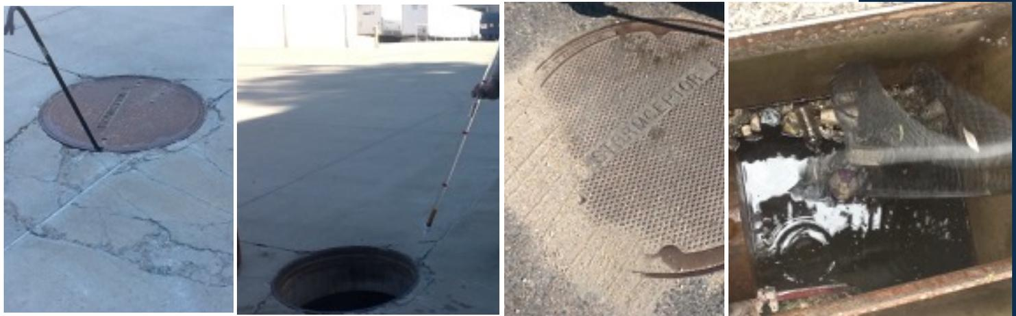
Proprietary device inspection utilizing "Sludge Judge" monitoring tool for sediment assessment on a Stormceptor Unit
