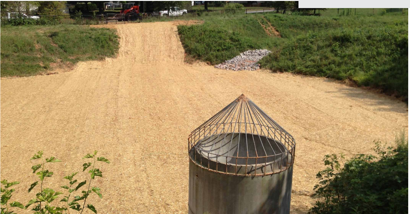
Sediment and Cattail removal at RETENTION POND
