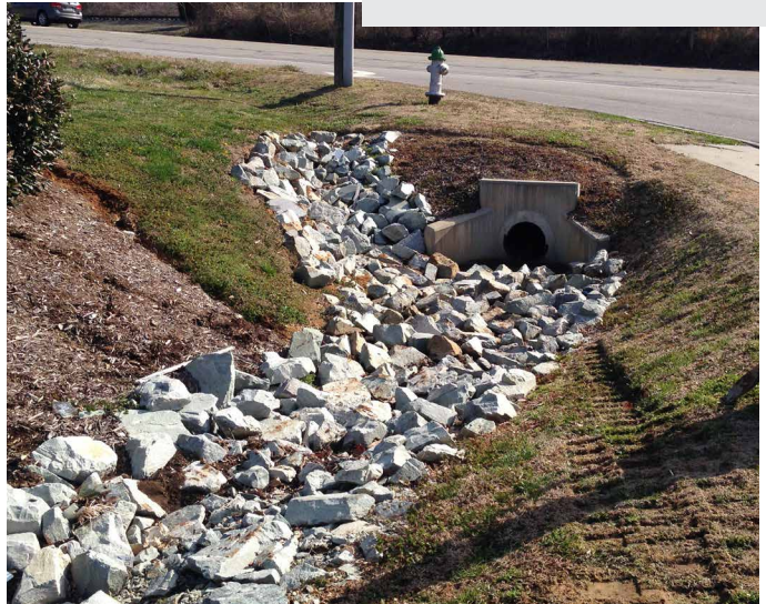
Repair at riprap SWALE
