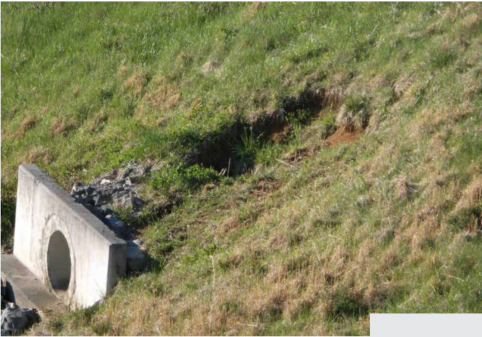
Pipe displacement at RETENTION POND
