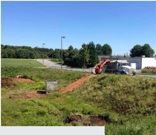
Sediment removal at bottom of DETENTION BASIN
