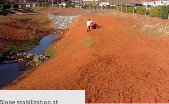
Slope stabilization at RETENTION POND
