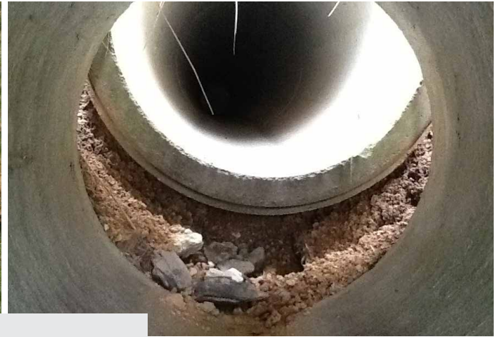
Pipe displacement at RETENTION POND
