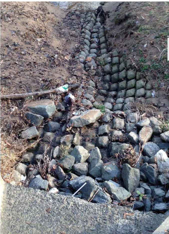
Inlet apron repair at SWALE
