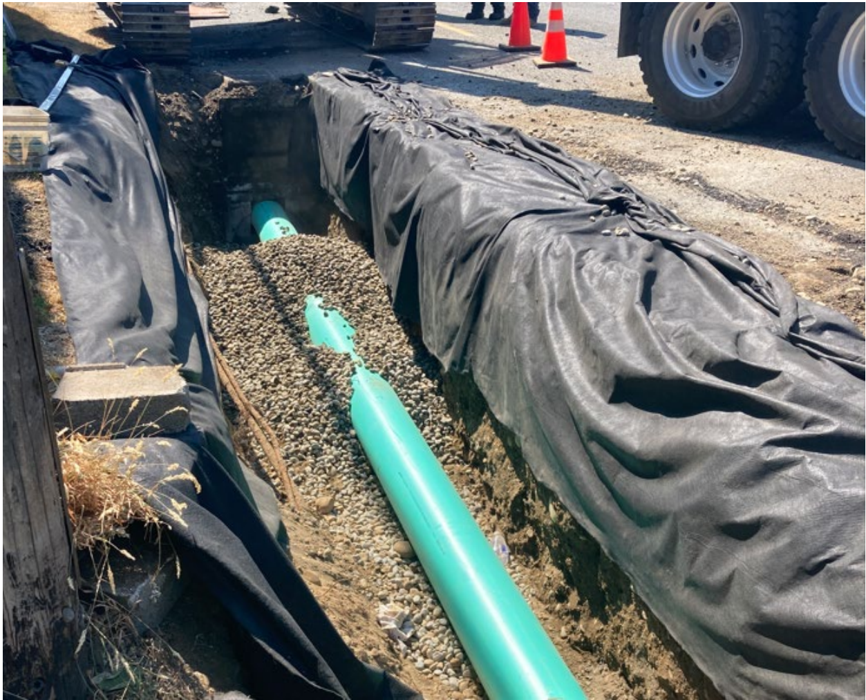
Installation of S Olympic Infiltration Gallery
