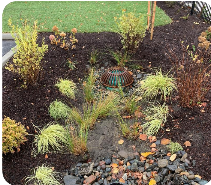
New Bioretention Facility at the St. Helens Village Apartments Completed in 2022
