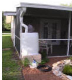
Figure 3.5-1 Rainwater Harvesting with a Rain Barrel
