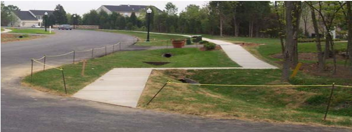
FIGURE 4-9 Recently Constructed Grassed Swale in Residential Area, Pembroke Woods Subdivision in Emmittsburg, MD (Courtesy of Mike Clar, Ecosite, Inc., Columbia, MD)
