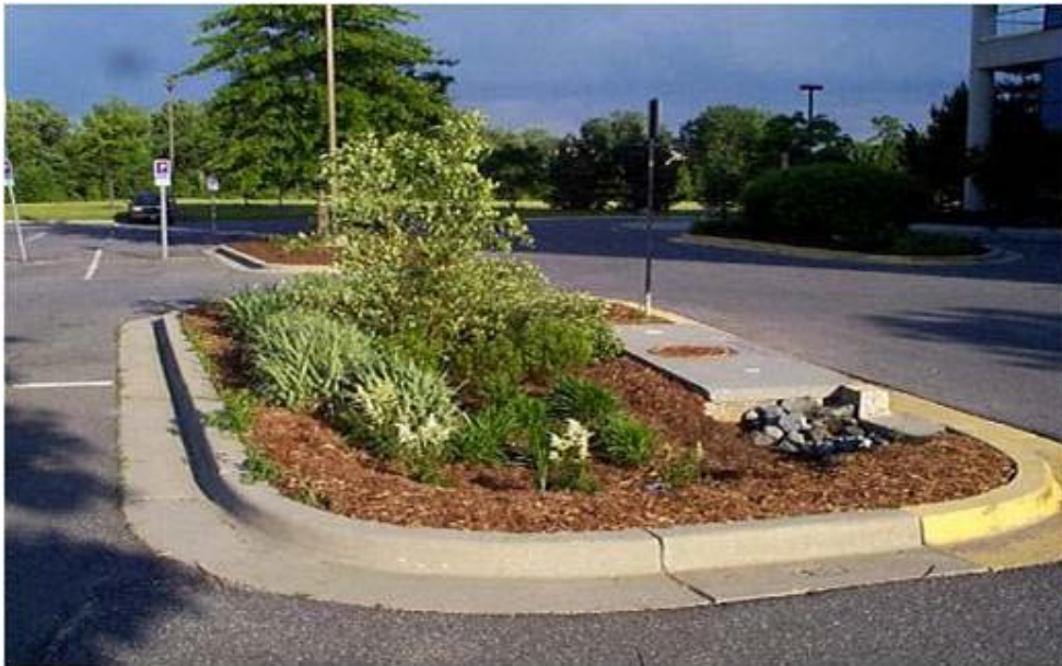
FIGURE 4-3 Bioretention in Parking Lot Island
