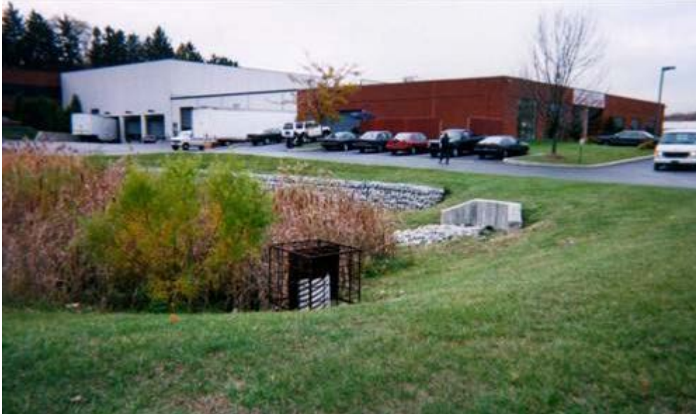
FIGURE 4-29 Dry Extended Detention Basin with Shallow Marsh
