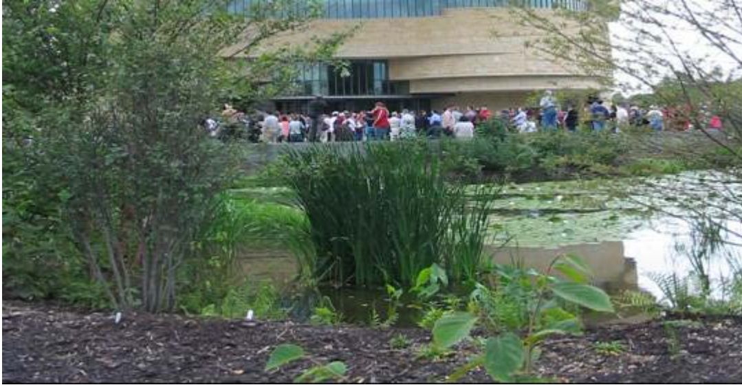
FIGURE 4-1 Constructed Wetland, National Museum of the American Indian in Washington, D.C. (Courtesy D. Medina)
