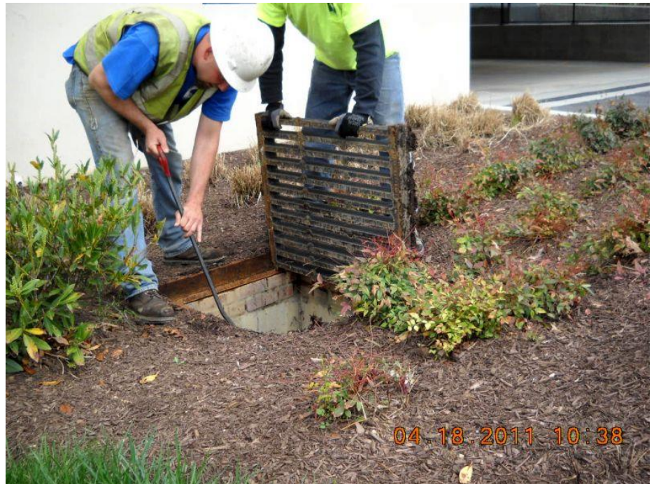
Figure 9-1: Bioretention Clean Out (source: Stormwater Maintenance Consulting)
