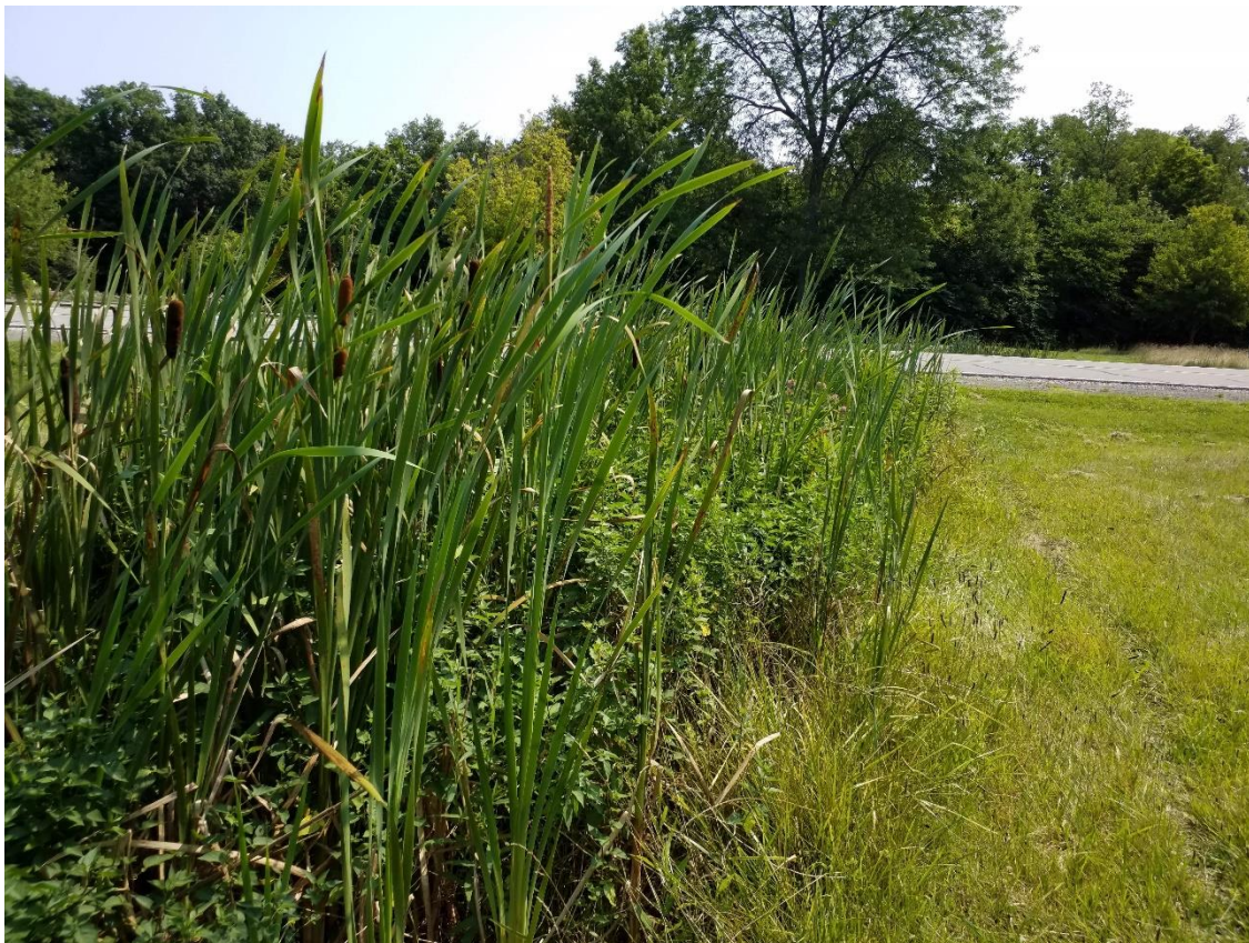
Figure 7-2: Swales can be used along roadsides and parking lots to collect and treat stormwater runoff (source: OHM Advisors)
