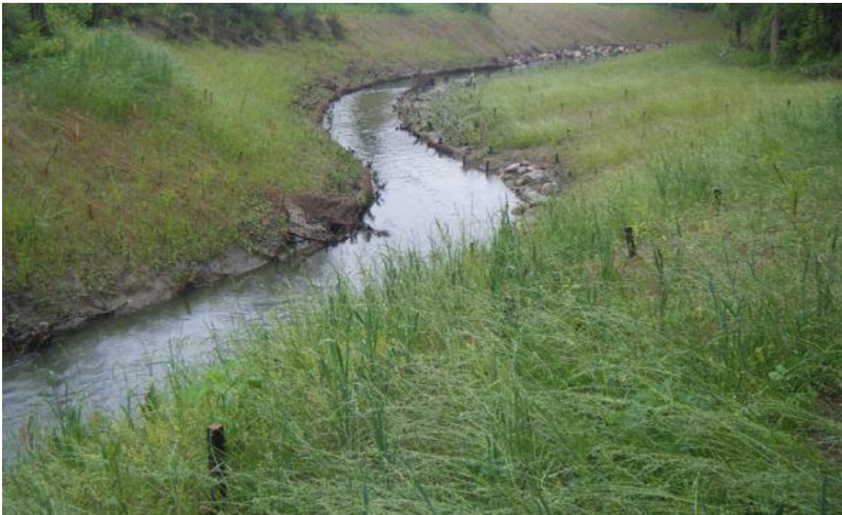
Figure 7-4: Streambank Stabilization after Construction (source: OHM Advisors)
