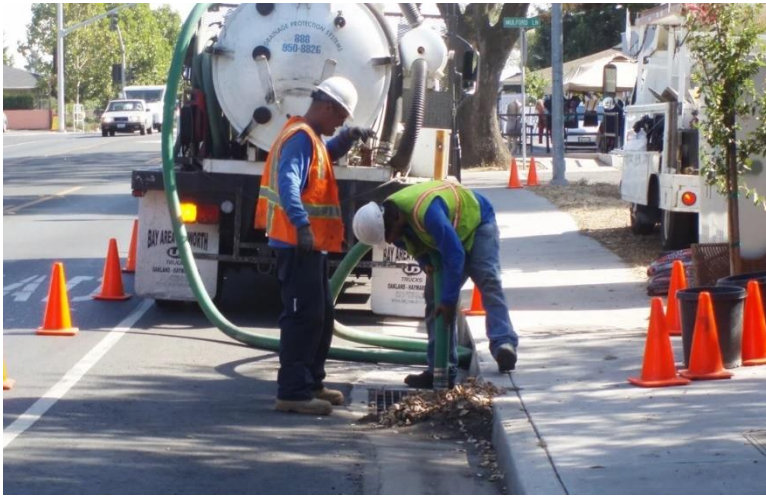
Figure 9-2: Closed Conduit Maintenance (source: CRH Building Solutions)
