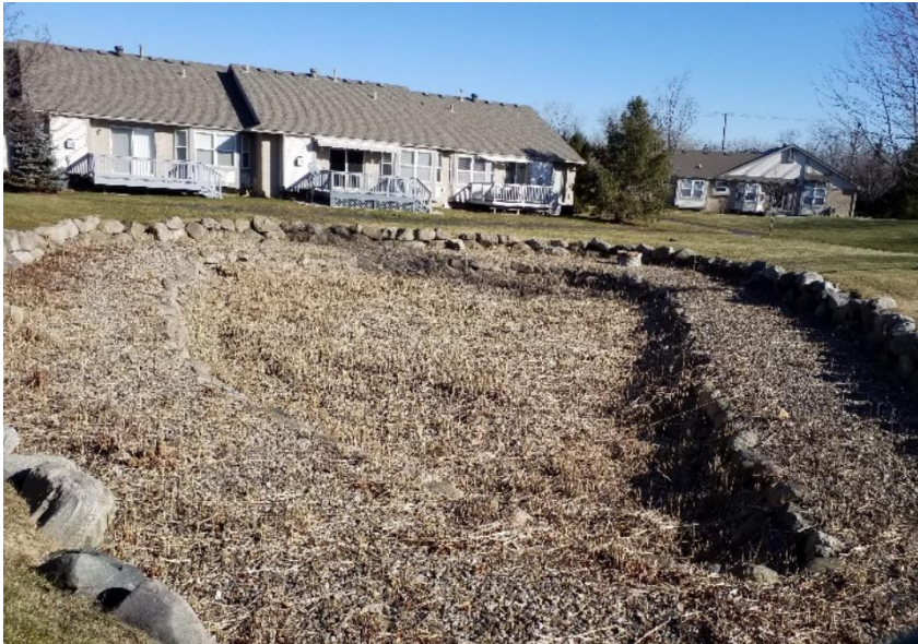
Figure 8-3: Dry Detention Basin (source: OHM Advisors)
