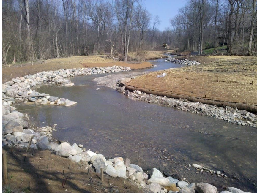
Figure 7-3: Streambank Stabilization During Construction (source: OHM Advisors)
