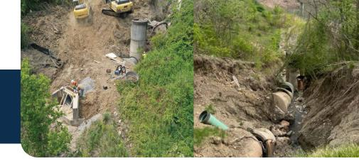
water rushed along the slope washing out sediment and the lower pipe sections. Erosion is an exponential problem and will worsen quickly. With combined flow now released down the slope, washout was significant.
